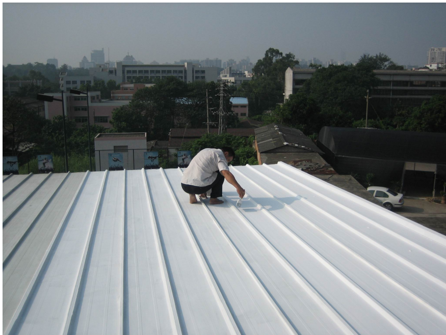
Painting the rooftop
